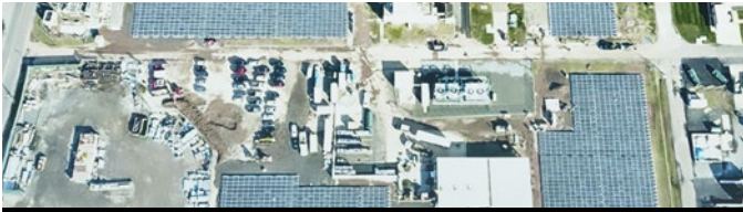
3.2 MW Brownfield Linden, NJ
